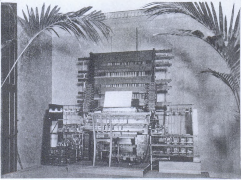
Fig. 32 (above). The Keyboard at Telharmonic Hall. (New York Electric Music Co., Telharmony , New York: The Company, late December 1906, 4)
