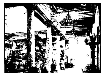
Main Corridor, Palm Room
